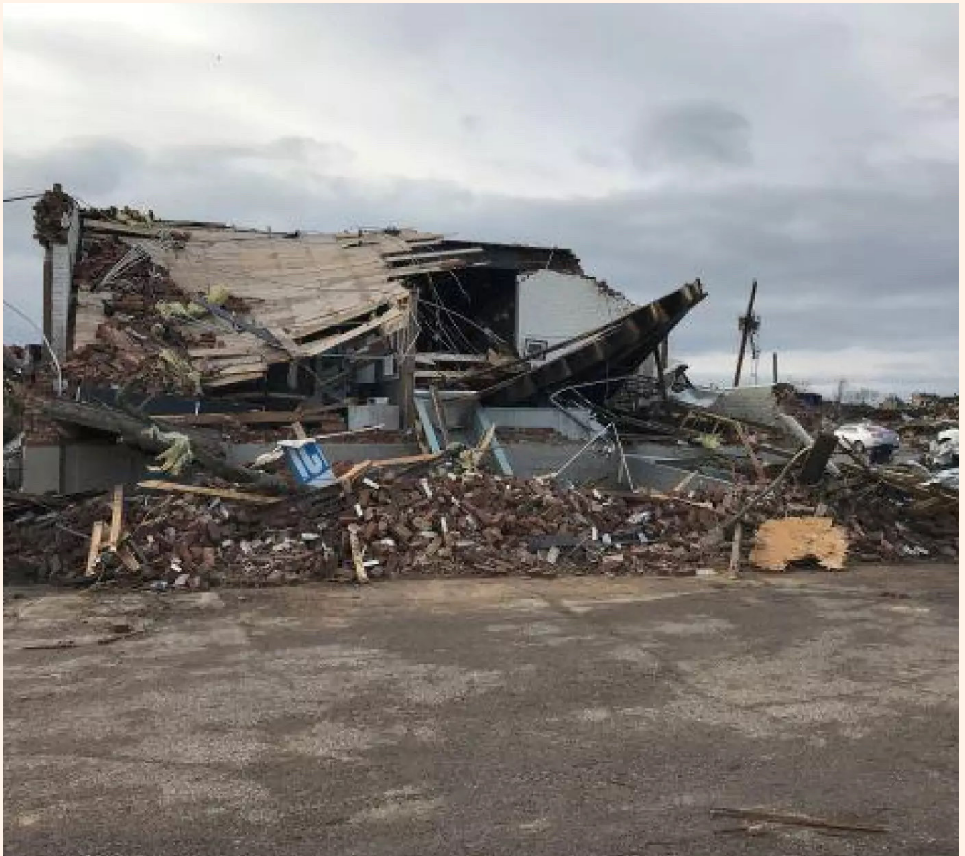
Credit: Ice House Gallery After the Tornado (Gunn 2021)
