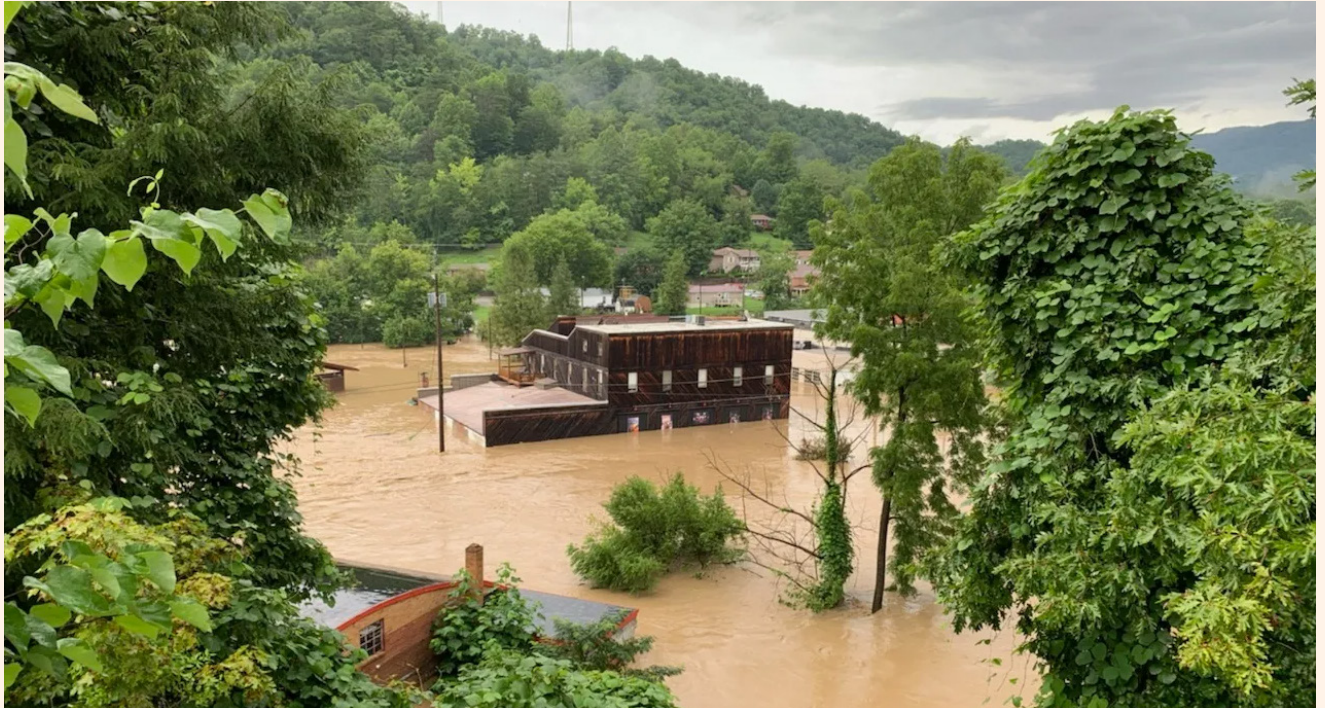
Credit: Appalshop's Madison Street Building in Floodwaters (Appalshop 2022)
